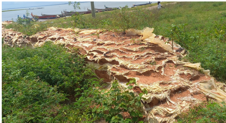
Figure 8: Sandbags to break shoreline change and floodwaters at Pitiko Source: Field Survey (2022)
