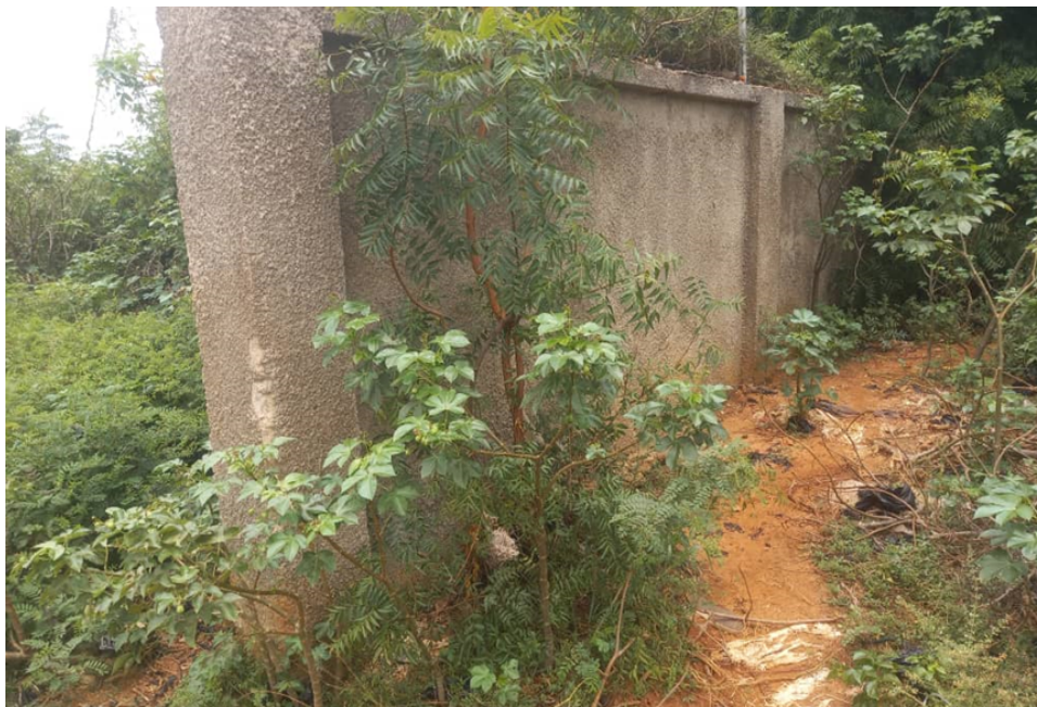
Figure 9: Retaining Wall in Adawso along the Afram River
